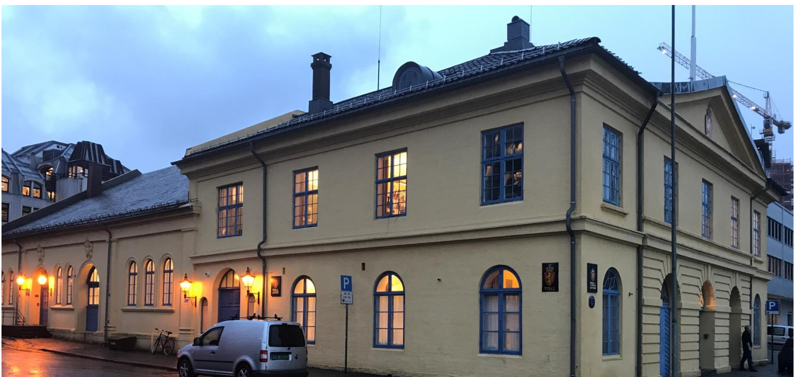
Outside view of the property Vestre Strandgate 21, Kristiansund, where the Customs Authority is tenant.
